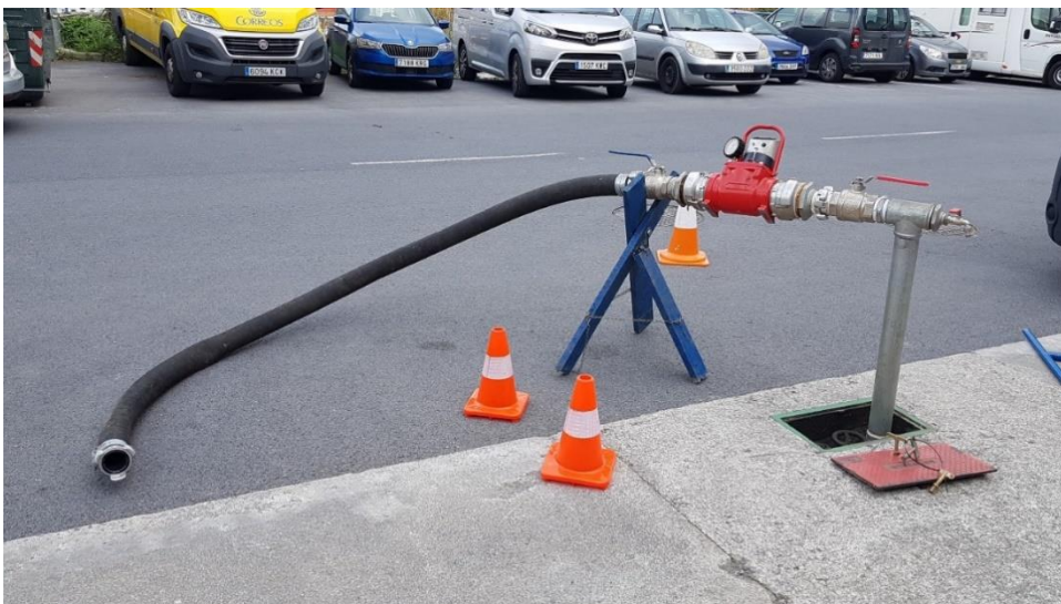
Illustration 3. Hose faucet with stand-pipe attached
